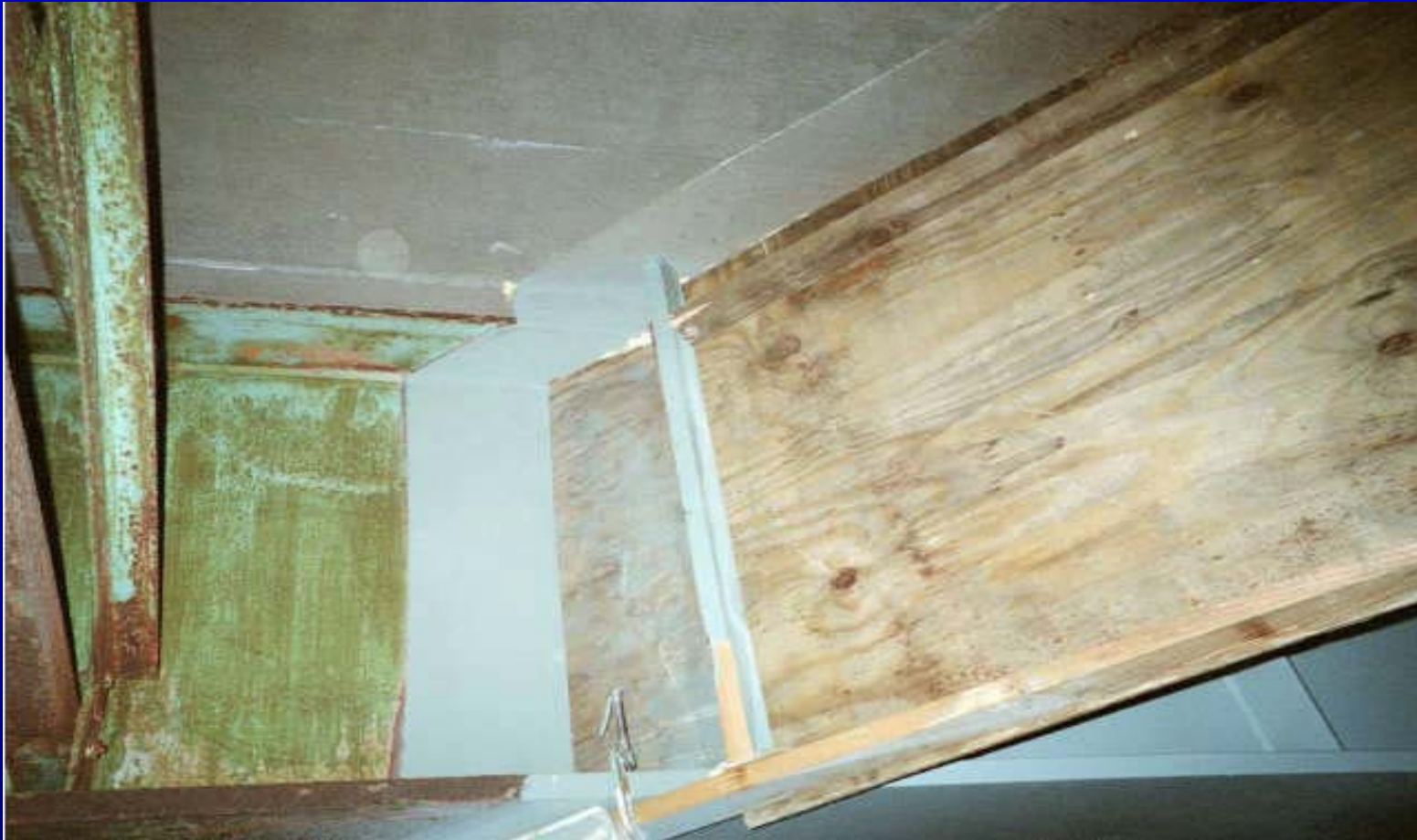
Bulkhead in place for overlap area
