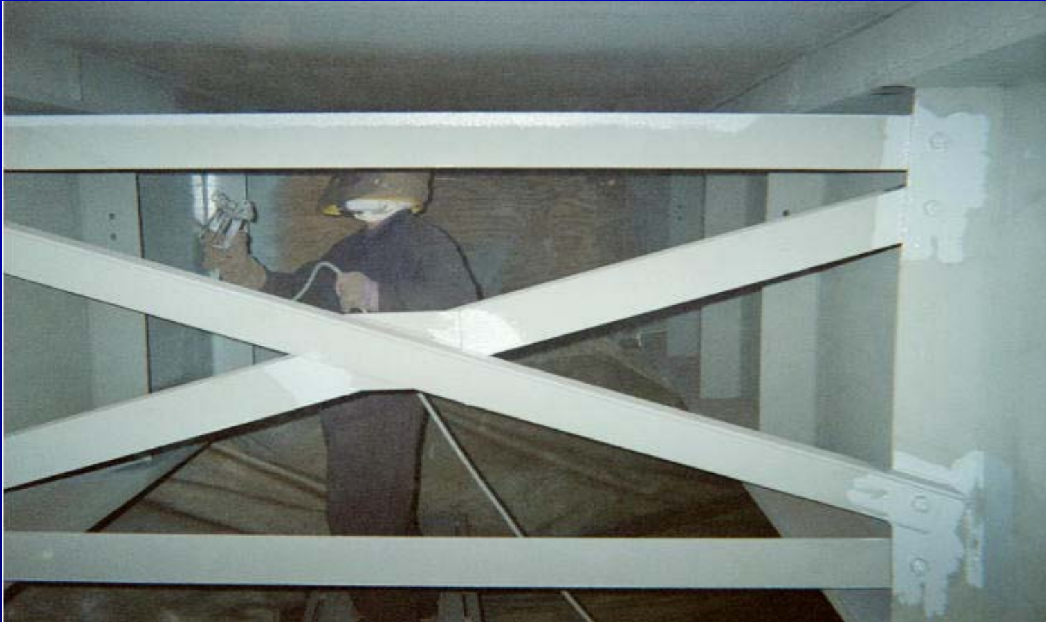
Spraying inside containment
