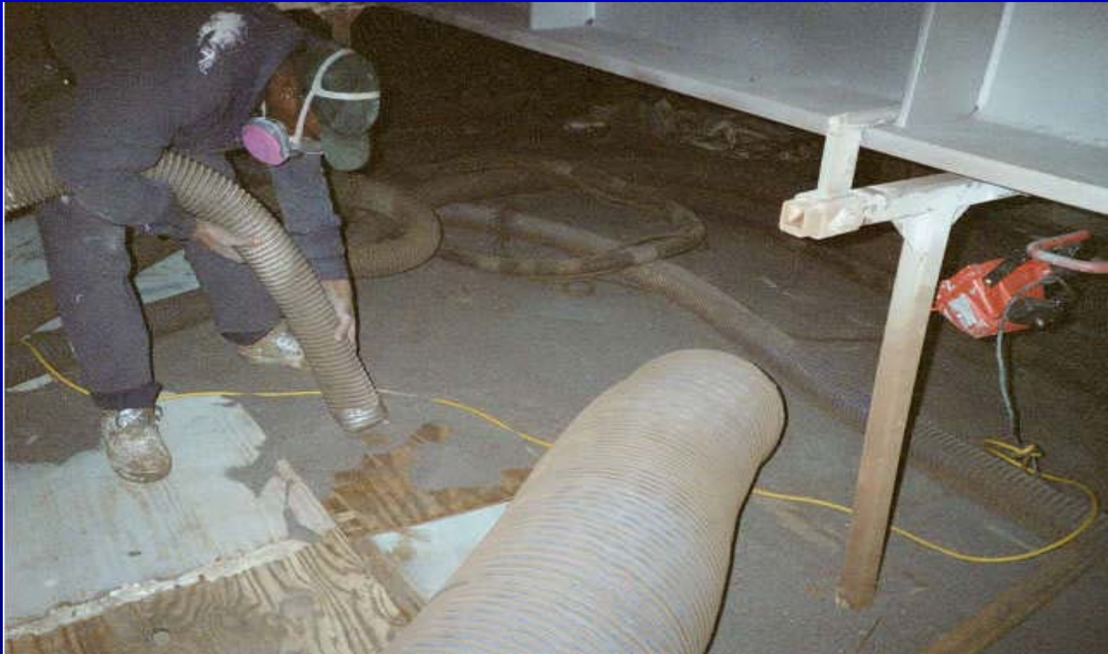
Vacuumping abrasive off floor in a traditional containment
