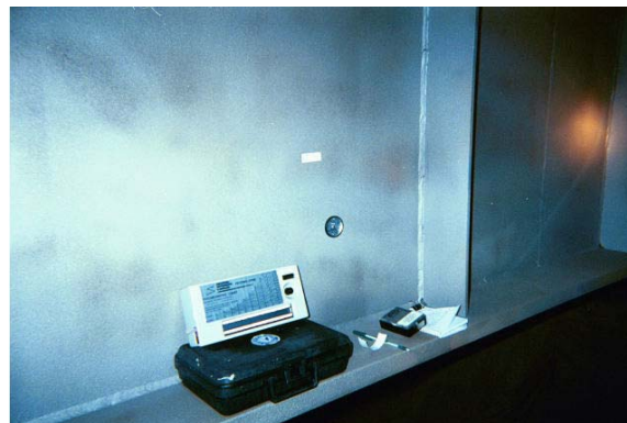
Blast cleaning and profile testing
