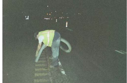
Vacuum spent abrasive in fixed containment
