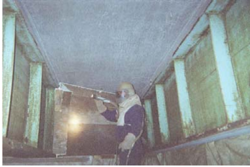
Mobil containment, good blast cleaning access
