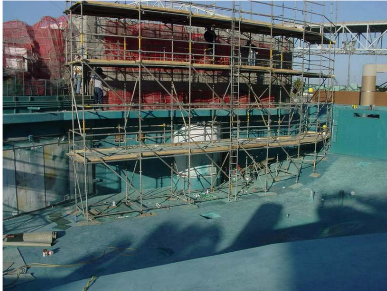
Figure 2: Scaffold Erection in Coating Application Area
