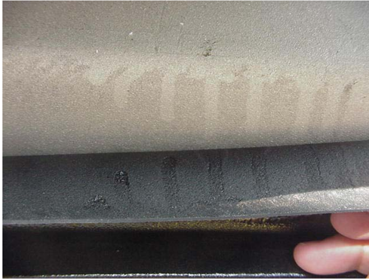
Figure 4: Delamination of Polyurea of Non-removed Soluble Salt Treatment
