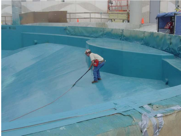
Figure 8: Spark Testing of a Polyurea Lining Project
