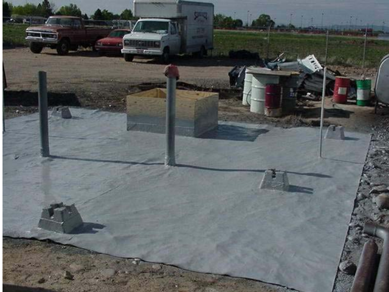
Figure 1: Mock-up Area for Landfill Lining Application
