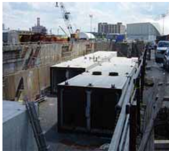
Two of three binocular immersed tube tunnels.
